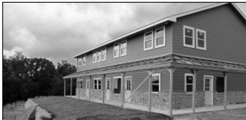
C3 OFFICE, MAILROOM and MERIT STORE nearly complete!
